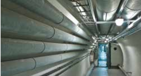
Bundesbank-Bunker, Cochem, Mosel-Saar
