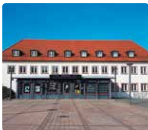
"Stadthalle" Civic Center, Landstuhl
