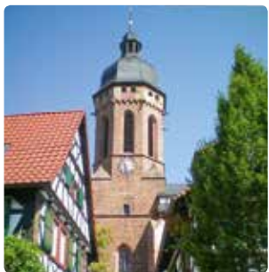
St. Georg's Tower, Kandel
